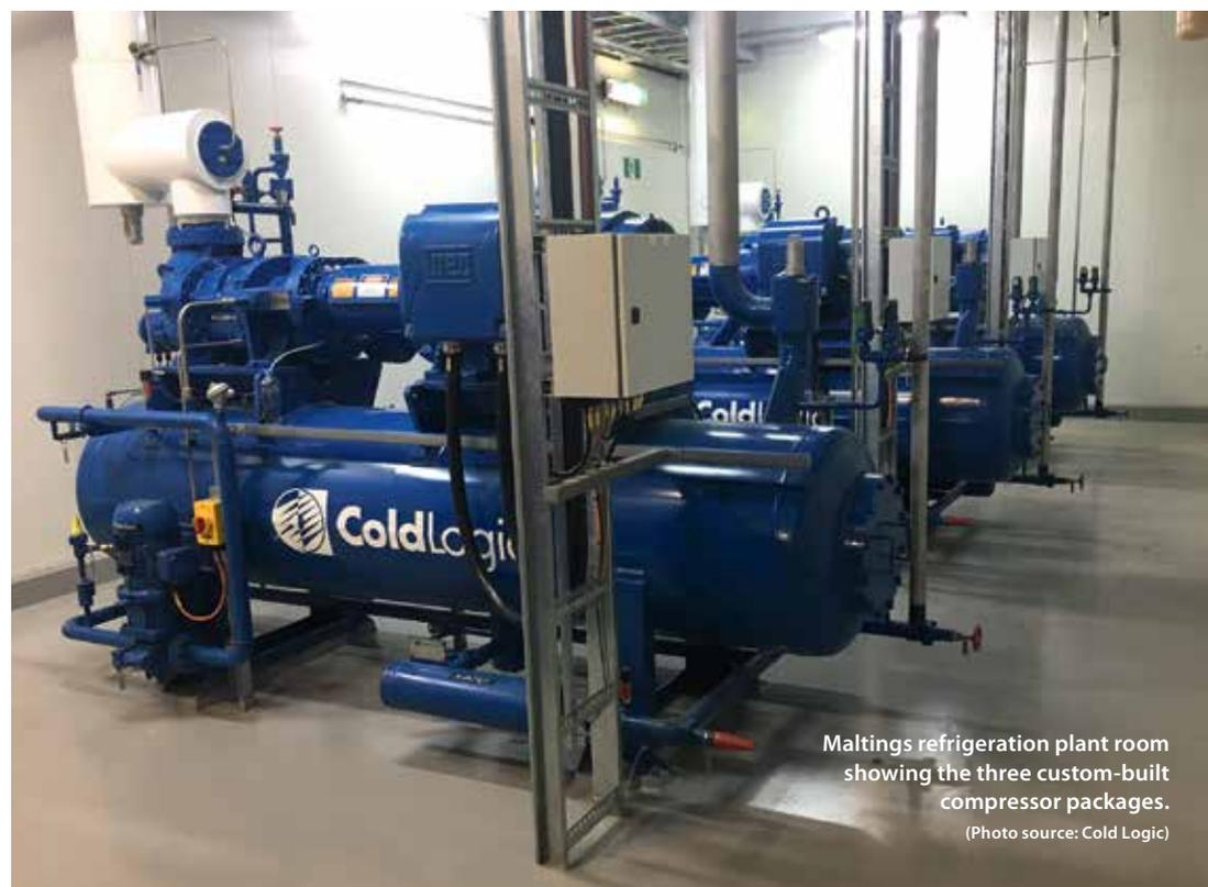
Maltings refrigeration plant room showing the three custom-built compressor packages.
