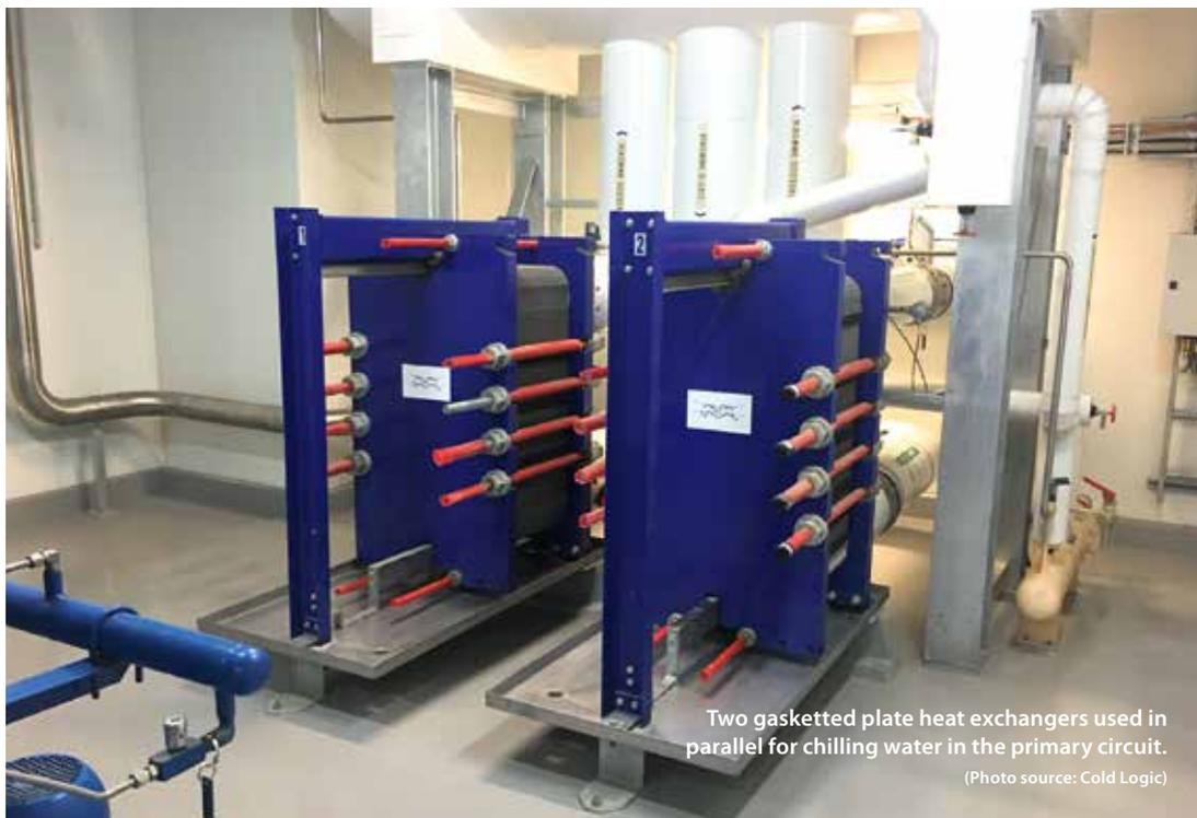
Two gasketed plate heat exchangers used in parallel for chilling water in the primary circuit.
