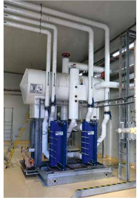
Inside the plant room showing the low pressure surge accumulator and plate heat exchangers.
