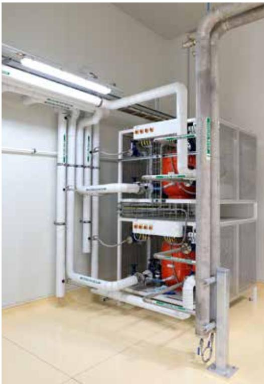
The ELK unit that controls the tempered water supply to the conches.
